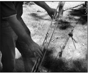
Step #3 Squeeze the strand together at the cross over mark and wrap the leg of the GUY-LOCK that is on top first. Wrap this leg completely until the rod ends are snapped in.
