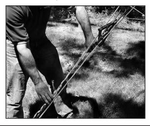
Step #4 Next, gently squeeze the strand together at the color code location. Wrap the second leg on the tail side of the strand, wrapping toward the hardware.
