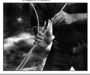
Step #7 To complete the installation, cut the excess strand at the desired location and secure tail to the main down guy.
