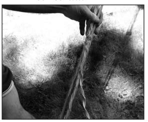
Step #5 Finish wrapping the second GUY-LOCK subset until the rod ends are completely installed.
