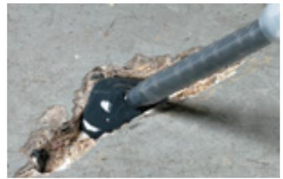
Nozzle automatically and precisely meters, mixes, and dispenses two-part urethane formulation. Apply material precisely where needed to conserve material.
