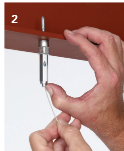
2 Push cable wire up through the bottom of KwikWire Hanger
