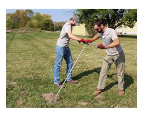
NOTE: When installation is complete, make certain that the eye of the anchor is in the correct position for guying before removing the installation tool from the anchor.
