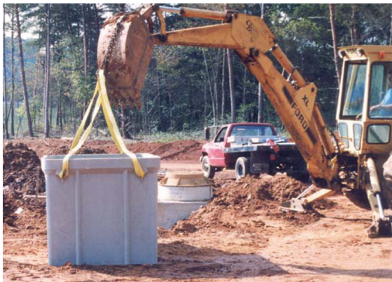
Lift and position enclosure with backhoe.
