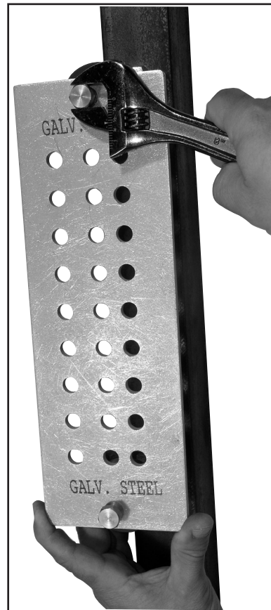
Insert torque shear head bolts. Tighten bolts until heads shear off.
