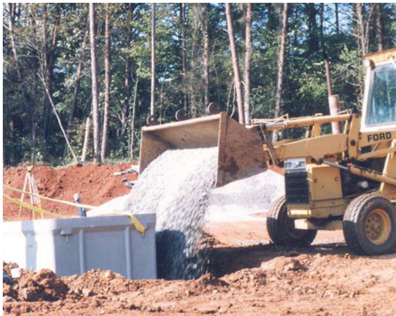
Place gravel in the enclosure and around the side. Lift enclosure to let gravel run underneath.
