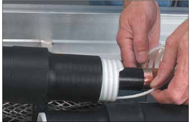
2. Position splice and unwind core
