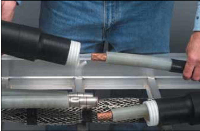
1. Prepare cable and make connection. Position 3M™ Cold Shrink Silicone Rubber Splice QS-III components
