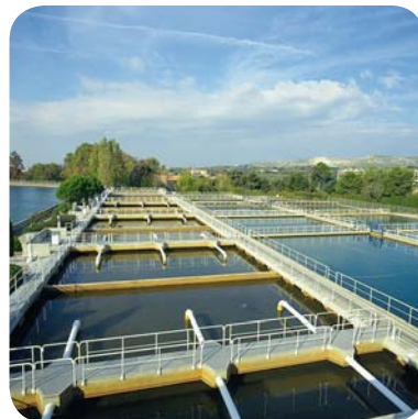
Water treatment application
