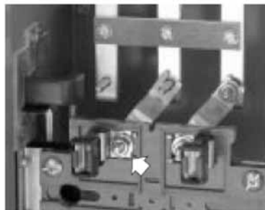
Step 4: Slide "Z" connector up to engage stud on B \phi vertical bus.
