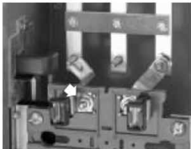
Step 2: Loosen hex nut from A \phi line side meter socket jaw and slide "Z" connector down to free connector from stud.
