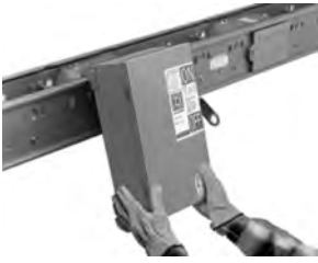
Figure 111 - Plug-In Device Mounting Example
