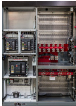
Main with Feeder Section
