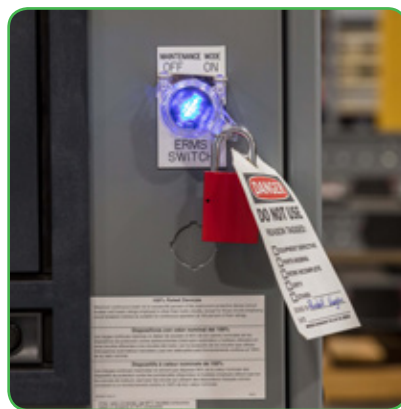
ERMS Switch with Lockout Tagout
