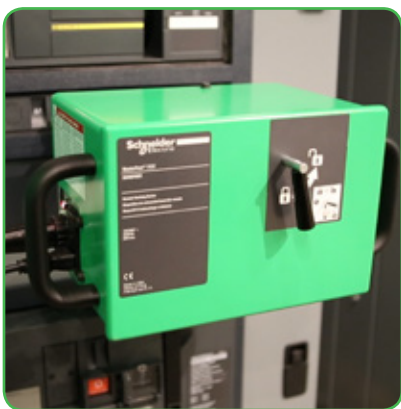
Remote Racking Device
