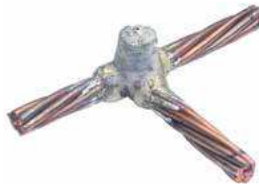
Acceptable. The presence of water/moisture in conductor strands or mold indicates that one or both were not properly dried. Although the riser is porous, the weld is solid. The degree of porosity is not sufficient to reject this connection.
