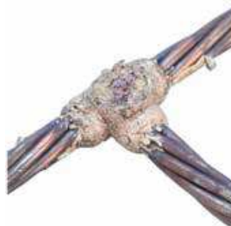
Reject. Excessive water in cable strands and/or mold.
