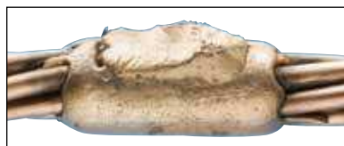
Fig. 29 Completed Cadweld connection.
