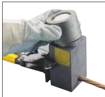
Fig. 22 Place the graphite Cadweld Exolon cover onto the mold, with the larger side facing down.
