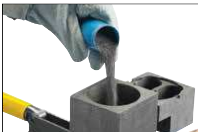
Fig. 20 Quickly pour the loose welding material powder into the mold.
