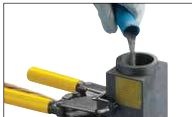
Fig. 21 Pour the loose welding material powder into the Cadweld Exolon mold.
