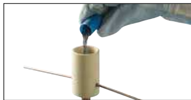
Fig. 11 Pour the loose welding material powder into the Cadweld One Shot mold.
