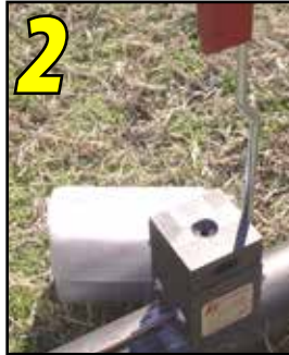
2 Position conductor and mold onto pipe.
