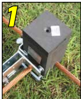
1 Position cleaned conductors in mold.
