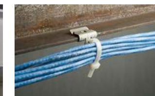
Cables from beam
