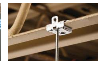
Threaded rod/chain/wire from beam
