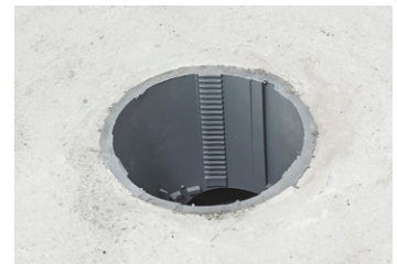
Cut box top level with concrete
