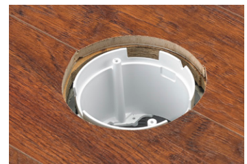
Install adjustable mounting cup and level with flooring
