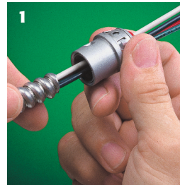
1 Snap fitting onto cable... twist clockwise
