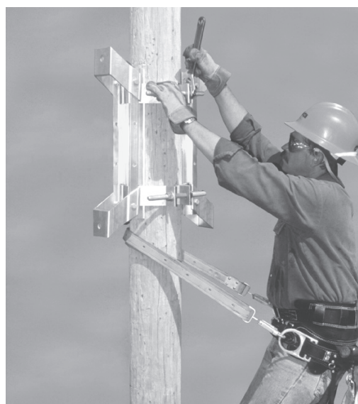
4. Tighten double-arming bolts. Mount transformers.
