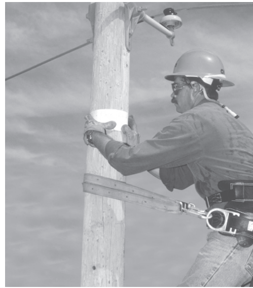
2. Using the tape provided, measure pole at the desired mounting height. Cluster mount will adjust to a wide variety of poles. Adjustment can be made at the ground.
