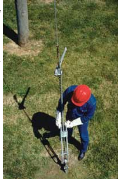
With 18" of adjustment, these Adjust-A-Grip deadend grips apply at the anchor end of guy strands.
