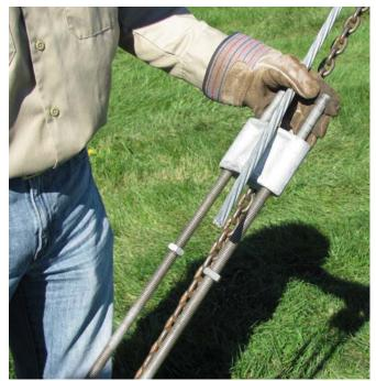
Cut the guy strand to the proper length. The cutoff point may be determined by sliding the socket onto the U-Bolt to the desired location then marking the guy strand (Left). Be sure to allow enough strand to extend at least two (2) inches beyond the end of the wedges (Right).
