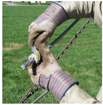
Position the two wedge halves around the guy strand at least two (2) inches from the end (Left), start the first rod subset by placing the color-coded end on the wedge. Allow the ends of the rod subset to extend approximately  $\frac{1}{4}$ - inch beyond the edge of the wedge (Right).
