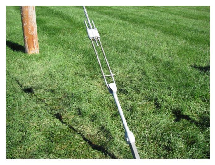
After the desired tension is attained, tighten all jam nuts. This completes installation if the tower height is less than 200 feet.
