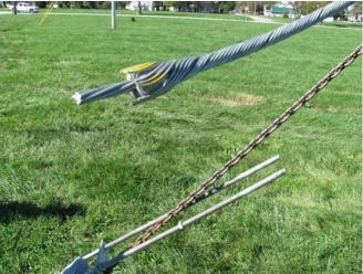
Complete the installation of rod subsets. Be sure the ends are snapped onto the guy strand (Left). Note that the formed ends spread symmetrically over the wedge (Right).
