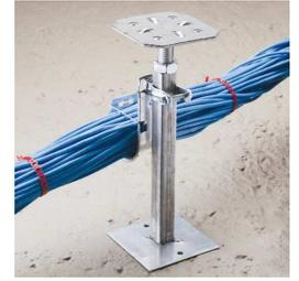
Cat HP assemblies are the fastest CATs in the Cat HP family by providing a high-performance J-Hook solution in a single assembly. They are ready to use right out of the box with a broad range of attachment methods. Cat HP assemblies are ideal for new construction or when the structural attachment requirements are well understood and installation speed is critical.
