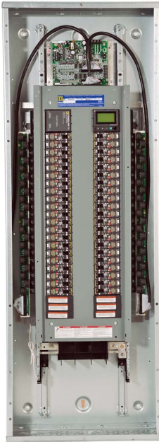
Powerlink Energy Management (EM) Lighting Control System
