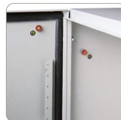
Welded studs for the ground connection.
