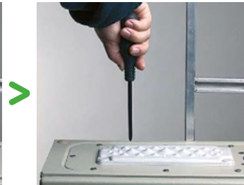
Make a small hole in the membrane.
