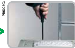
Make a small hole in the membrane.
