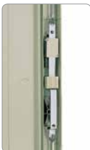
Detail from the internal locking system.
