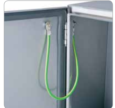
Grounding studs welded to the door and in the body.
