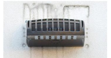
Example of retrofit not matching existing fixture footprint with unsightly wall stains.
