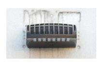
Example of retrofit not matching existing fixture footprint with unsightly wall stains.
