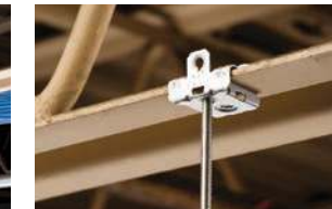
Threaded rod/chain/wire from beam
