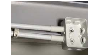
Conduits & electric box from beam
