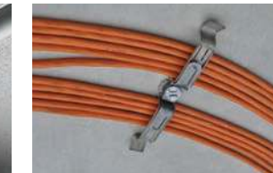
Cables from concrete ceiling/wall
