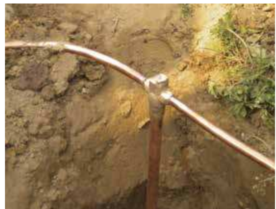
GT Cadweld connection
