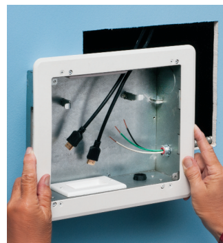
Install trim plate on box. Pull wire. Insert assembly into opening.
