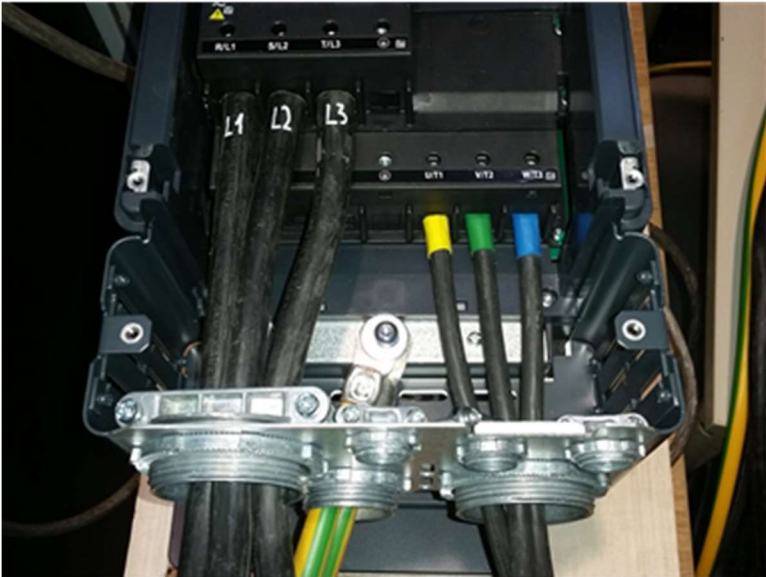
Figure 4 VFD Terminations
