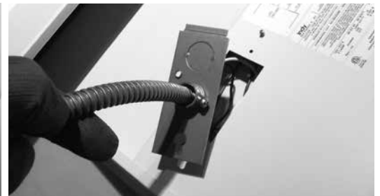
Step 3 Insert connector. Wire to fixture appropriately based on dimming requirements. See wire diagram on fixture.
