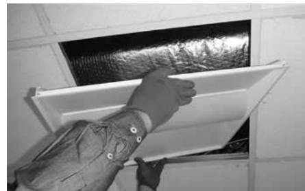
Step 5 Install troffer into grid.
