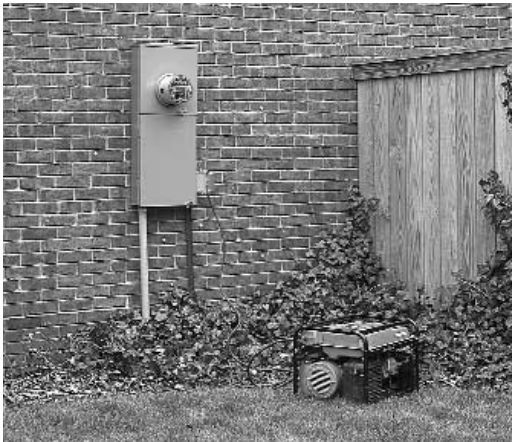
The SO2040M200S has provisions to accept our Standby Generator Kit, which provides easy switching between the main breaker and the generator-fed breaker.
