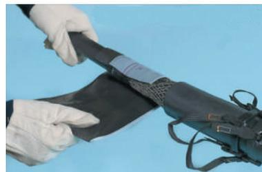
Applying sealing mastic
