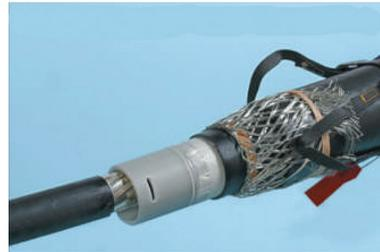
Support tube in self-ejecting mode
