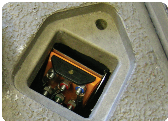
Bonding Harness Or Locate Wires
