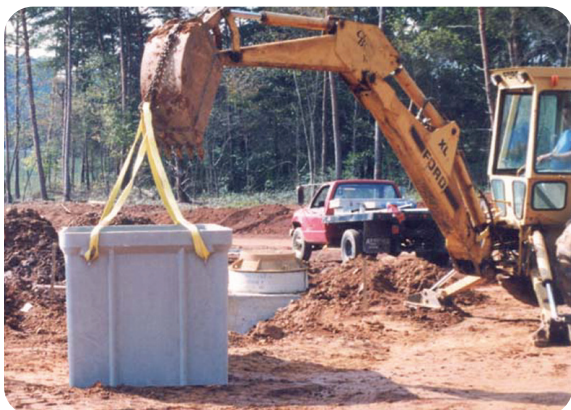
Lift and position enclosure with backhoe.
