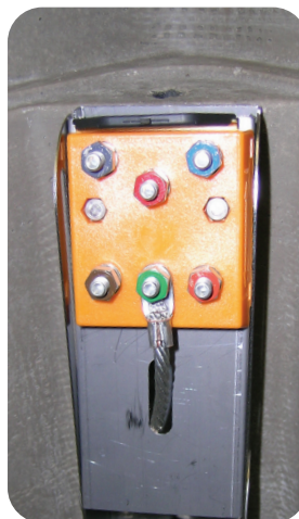
Test Station or Isolation Switch
