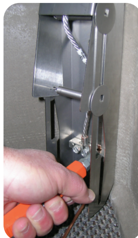
Test Station or Isolation Switch
