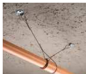
Attache de retenue universelle CSBURCxxxx – p. 33 CSBURCRxx – p. 34
