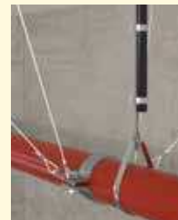
Pipe Rod Stiffener CSBRS1 – p. 36
