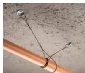
Universal Restraint Clip CSBURCxxxx – p. 33 CSBURCRxx – p. 34
