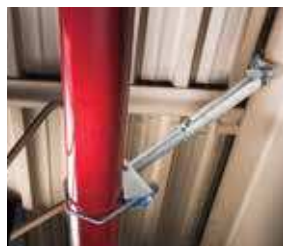
Lateral Telescoping Brace Assembly CSBTx – p. 31
