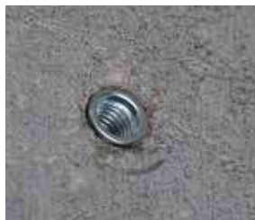
Branch Line Restraint Structure Attachment to Threaded Hole CSBBRS3MEG – p. 38
