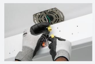
Optional quick-mount bracket allows direct installation to j-box without opening the fixture at all.
