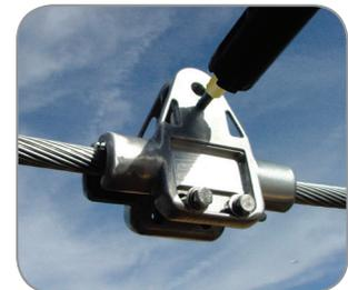
4. Once in position, rotate the "Hot Stick" (with Live-line Attachment Tool attached) in a clockwise direction until the HIBUS Suspension is fully closed
