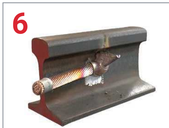
5 After reaction, open the mold and remove the expended steel cup – no special disposal required.
