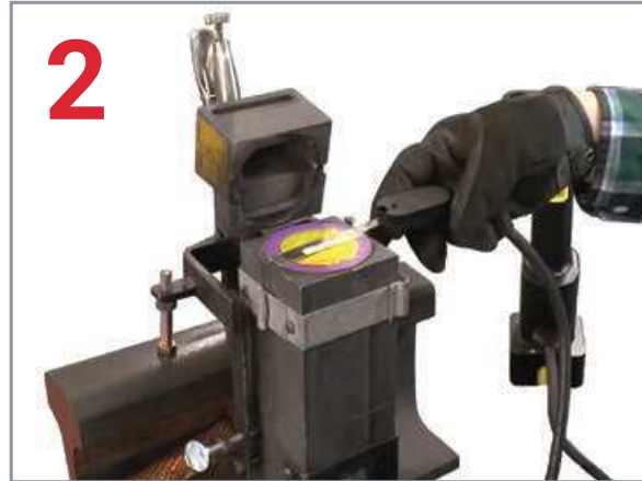
2 Attach control unit termination clip to ignition strip.
