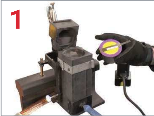
1 Insert Cadweld Plus cup into mold.
