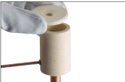
Fig. 12 – Place the cover on the top of the Cadweld One Shot.
