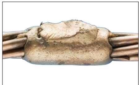
Fig. 29 – Completed Cadweld connection.
