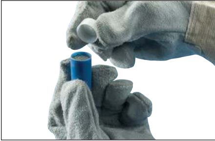
Fig. 10 – Next, take the tube of welding material included in the Cadweld One Shot package and remove the lid over the crucible.
