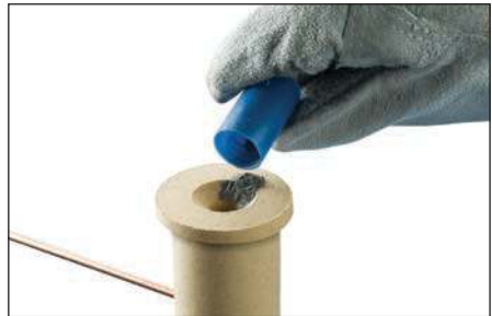
Fig. 14 – Pour the starting material onto the Cadweld One Shot cover.
