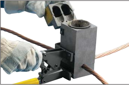
Fig. 21 – Remove the control unit connector from the ignition strip. Open the lid and remove the used Cadweld Plus cup from the mold.
