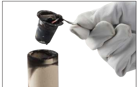
Fig. 14 – Remove and dispose of the used Cadweld Plus weld metal cup.
