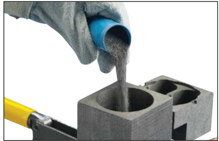
Fig. 20 – Quickly pour the loose welding material powder into the mold.
