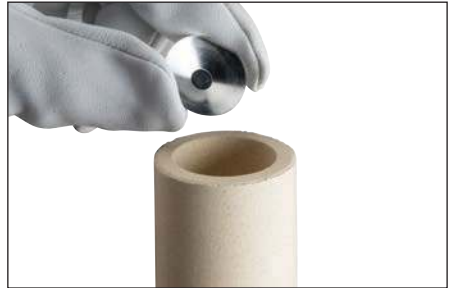
Fig. 8 – Place the steel disk into the Cadweld One Shot with the concave side facing up.
