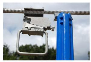
10) Slide interface along main wire and into the connector until it reaches the stop.
