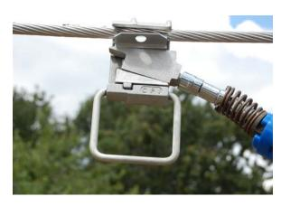
12) Use a universal socket stick and 3/4" socket to tighten bolt until Hex Head shears off. The bolt should break off at 110-130 INLBS (12-14 NM)
