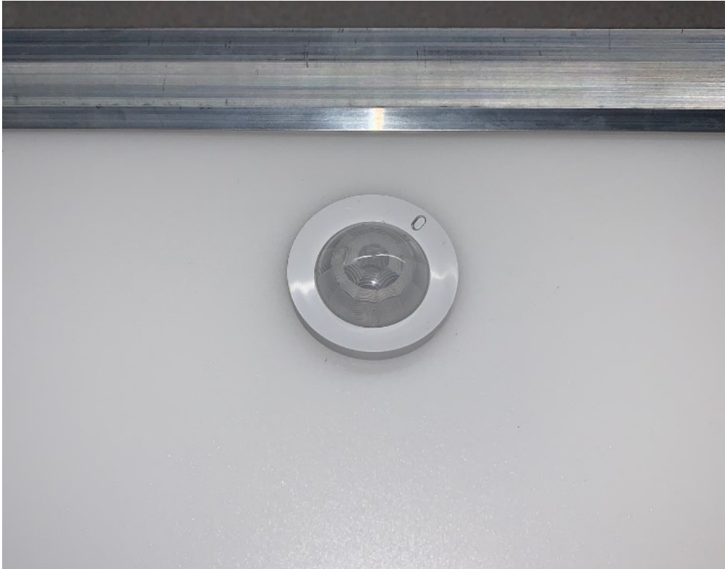
Figure 17: RES7 sensor optic snapped in place
