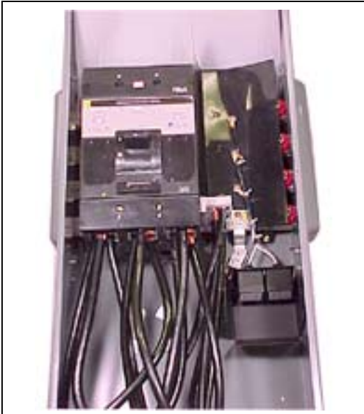
Figure 1: Secondary Surge Arrester
