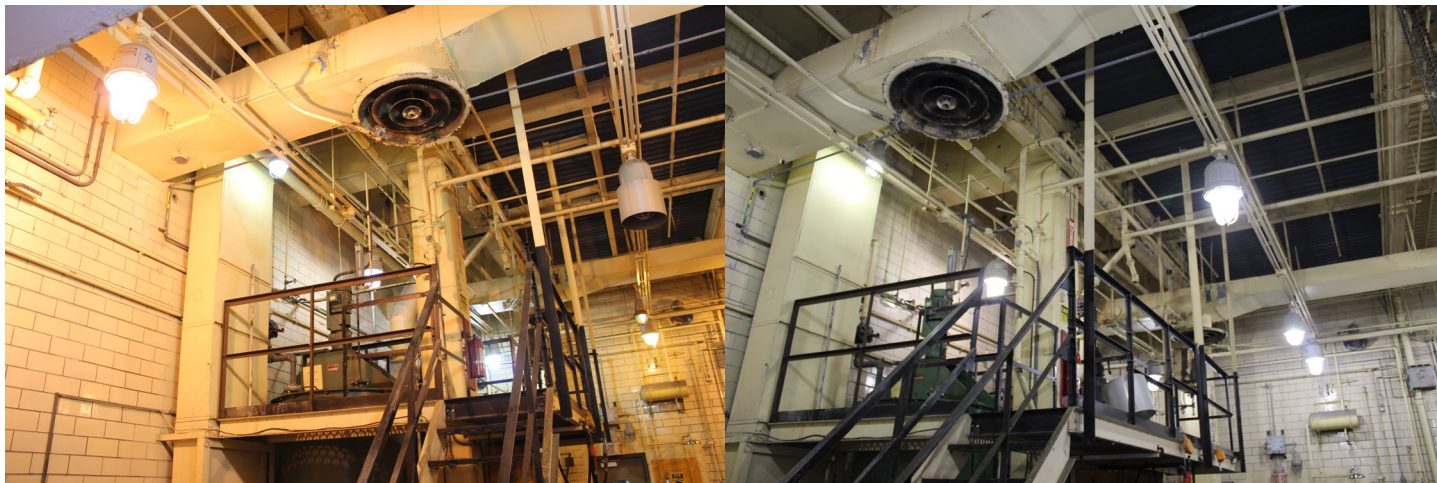
Before: 250W High Pressure Sodium Lamps
