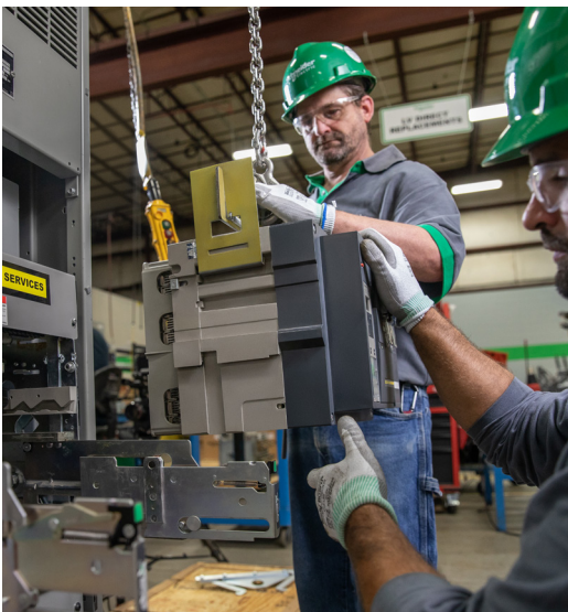
The switchgear structure, conduits, cabling and footprint are left intact, which saves time and money (above).
