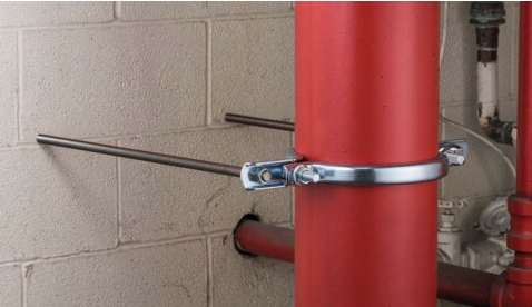
456 Malleable Split Ring Hanger for Copper Tube 456####CP
