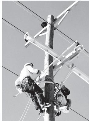
Two conductor covers lock together on a 13kV line where an insulator cover is not required.
