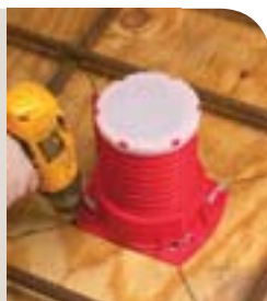
3. Secure to decking
