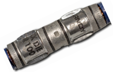
Completed Crimp Installation
