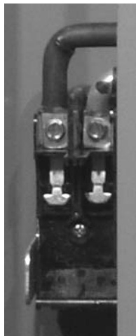
QO Plug-On Mounting Base
